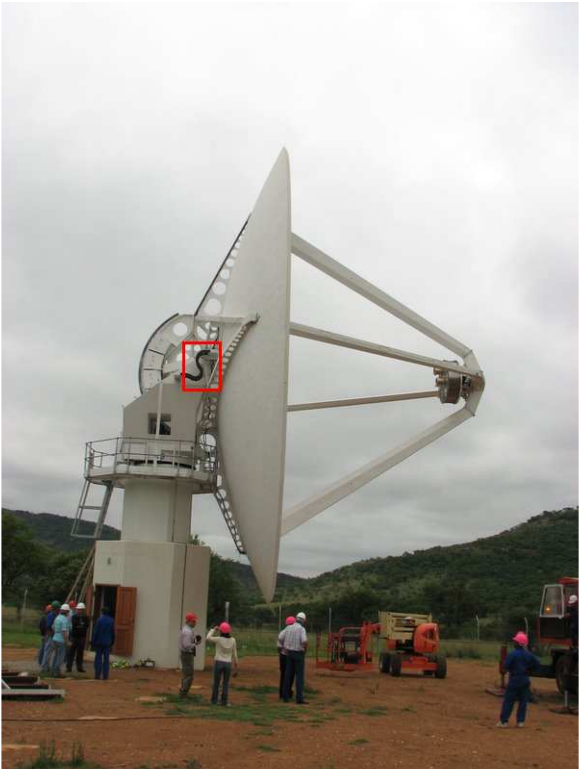
Figure B.2: Elevation cable wrap at a lower angle. The cable wrap at this lower dish angle position subjects the riser cable to more bending
